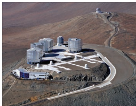
View from the south The European Southern Observatory's Very Large Telescope (VLT) in the Atacama Desert in northern Chile.
